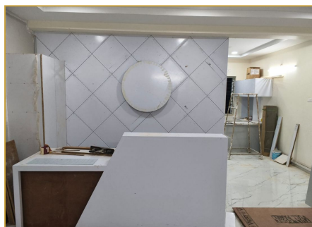
Reception feature wall under construction
