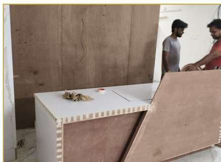
Reception counter joinery being assembled
