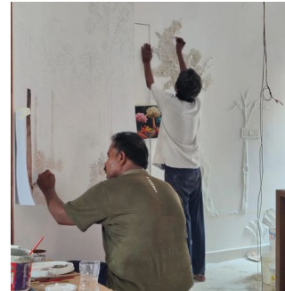
Hand-crafted textured mural being executed on site
