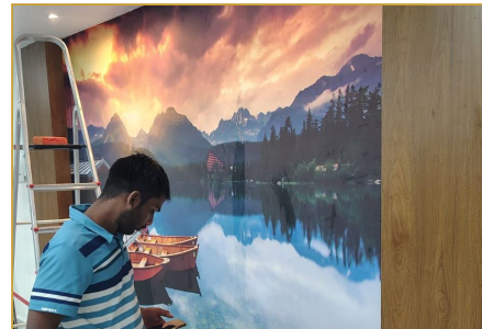
Mural panel installation
