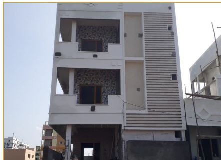
Completed residence — textured cladding elevation
