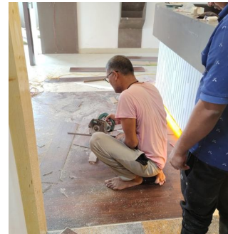
Laminate flooring cutting and installation
