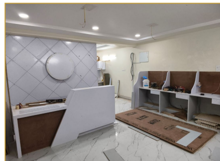
Reception counter and workstations in progress
