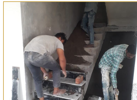
Granite staircase cladding
