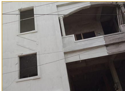
Arched balcony facade at finishing stage
