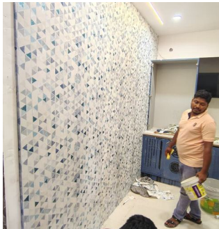
Mosaic tile feature wall installation
