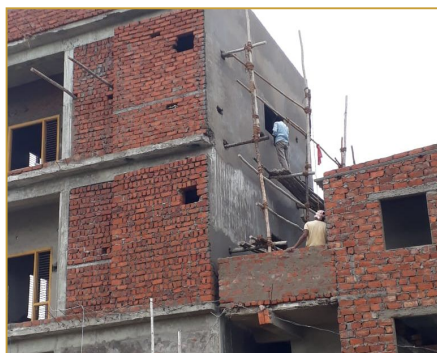
Civil construction — structure and masonry
